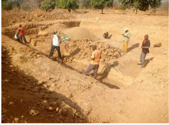
Mengukya community group excavating group farm pond
