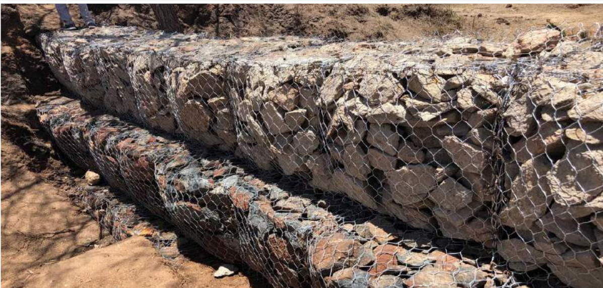
Rehabilitation work in progress at Musalabani rehabilitation site in Makueni county
