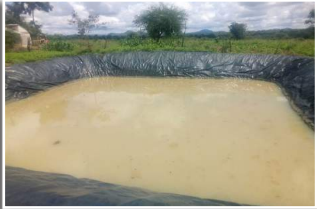
Mengukya finished farm pond measuring 396 cubic metre
