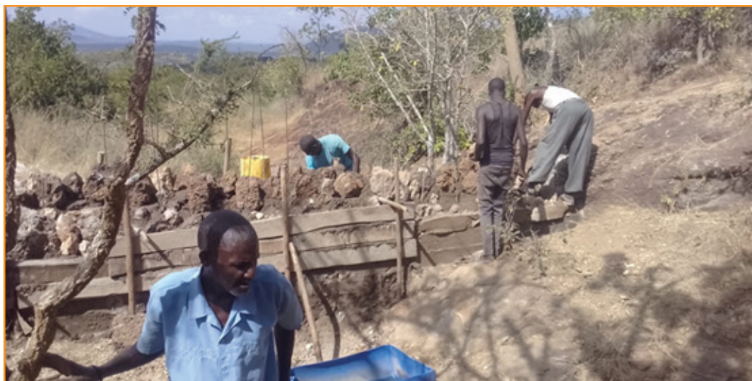
An individual community member within Ikolya watershed undertake construction of a sand dam across a stream for land scape restoration in Kilome Sub County-Makueni County
